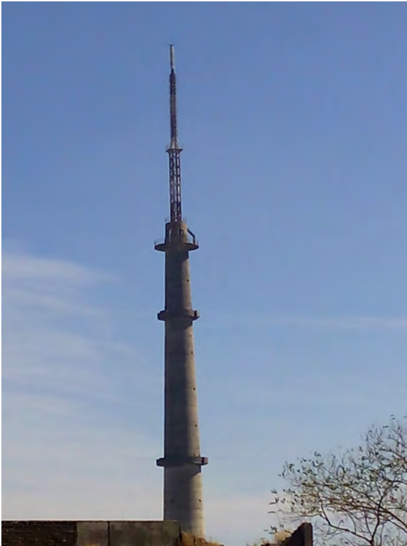
Transmitting Antenna Tower
