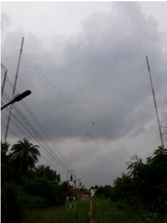
Transmitting Antenna Tower
