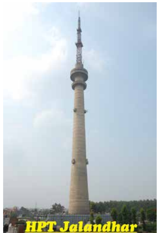
HPT (TV) Antenna Tower
